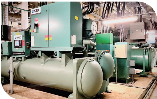
A total of six new heat exchangers and two new chiller units now serve the Cyberport community, saving 200,000kWh and 1,300,000kWh of energy, respectively. 目前共有六台新的熱交換器和兩台新的冷水機組為數碼港社群服務，分別節約200,000千瓦小時和1,300,000千瓦小時能源。
